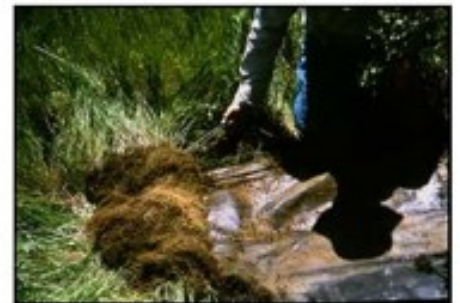
Sod growing on top fabric
